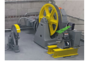
Elevator Rope Inspection
