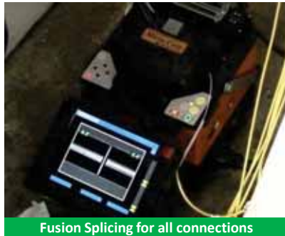
Fusion Splicing for all connections
