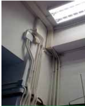
Special Fiber installation in congested conduits
